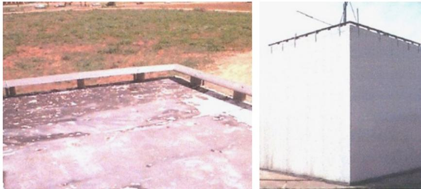
Fig. 9. Roof-edge fairing on the TTU Building (after Banks et al., 2001).
